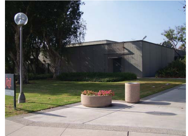
Figure 2-1: Half Dome building
