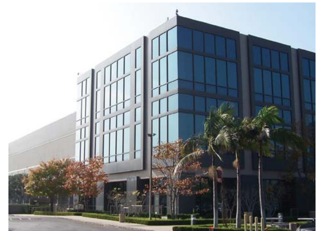
Figure 5-1: Existing TowerJazz Building
