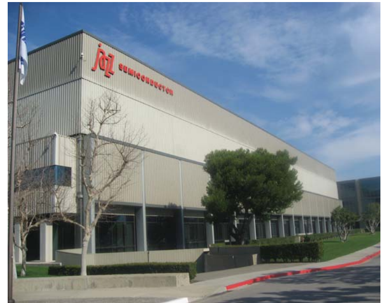
Figure 3-10: Existing TowerJazz Building
